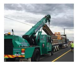
d) Ensure crane operator lowers the barrier(s) before traversing to increase load stability when getting in to position.
