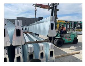
Forklifts are not to be used to load or unload barriers using the normal tyne method.
