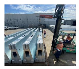
NOTE: There are on 10 barriers maximum on a standard semi-trailer bed. 2 x rows of 5 units.
